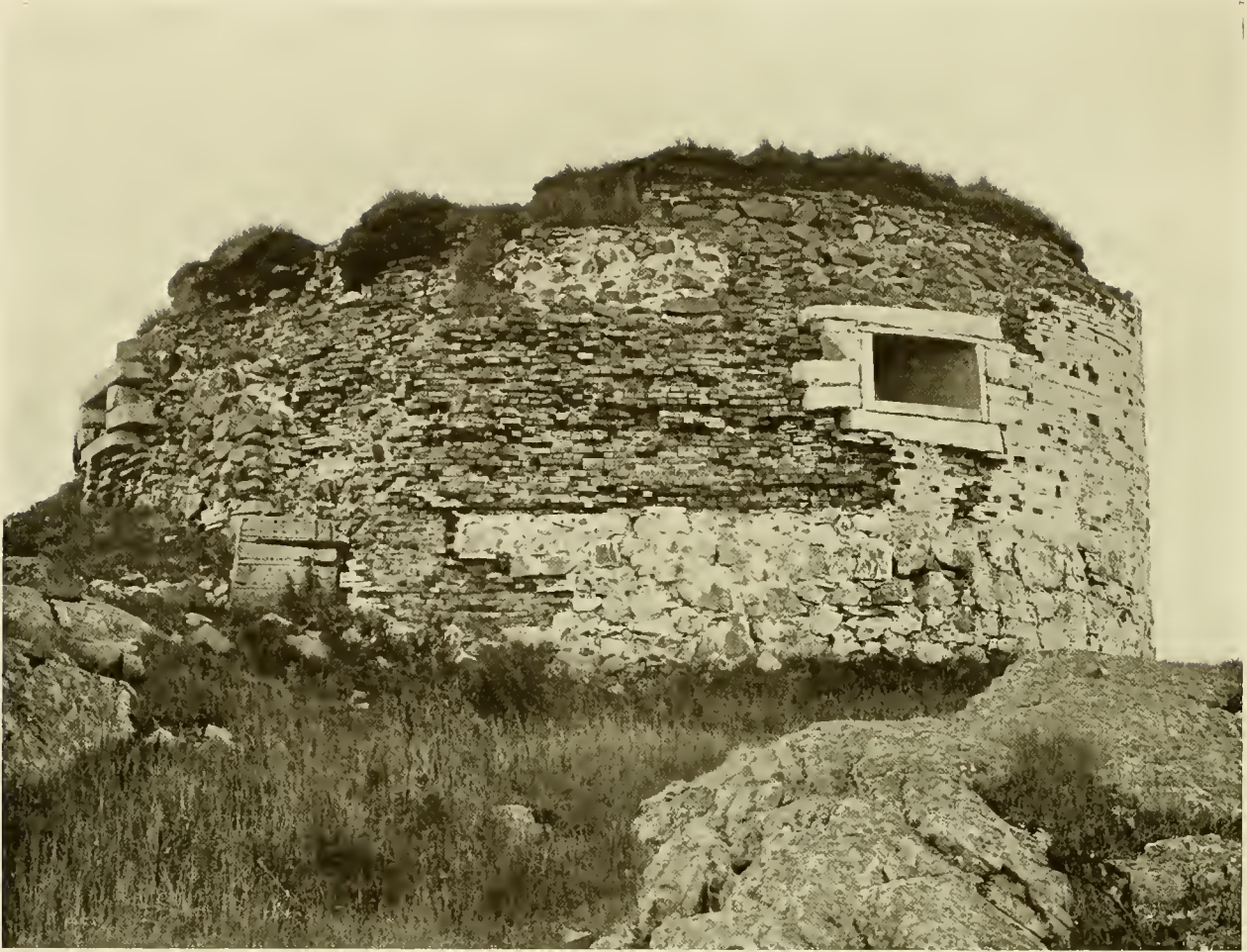
THE WALBACH TOWER, NEW CASTLE, N. H.
